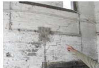
**Figure 4 Cracks due to Openings in Walls**
