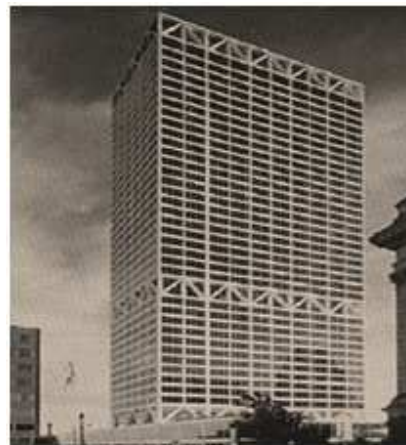
Fig. 9 Outrigger belt truss system
