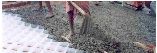
Figure 2 placing of zero slump concrete into cells during construction of a road
