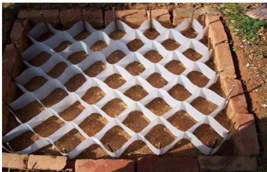
Figure 1 Laying of formwork of plastic cell over a compacted sub grade/sub base.
