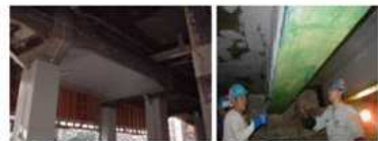
Fig 11. (a) Strengthening of Slab (b) Strengthening of Beam
