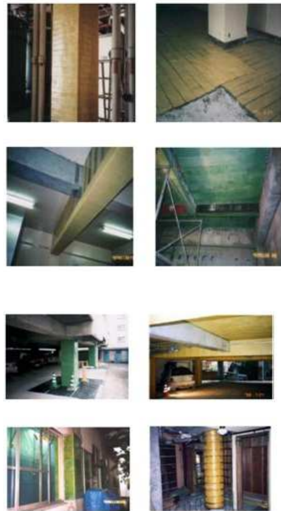
Fig 10. Applications of AFRP Sheets in Building Structures
