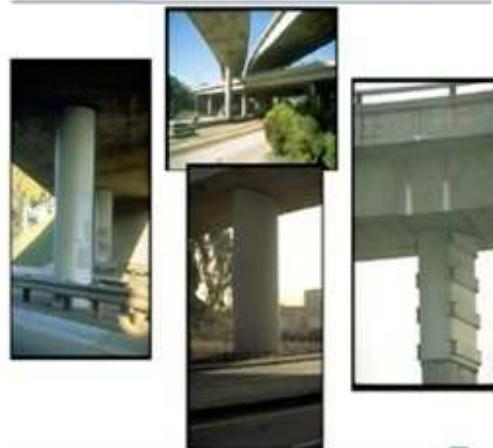
Jacketing: RC bridge piles
