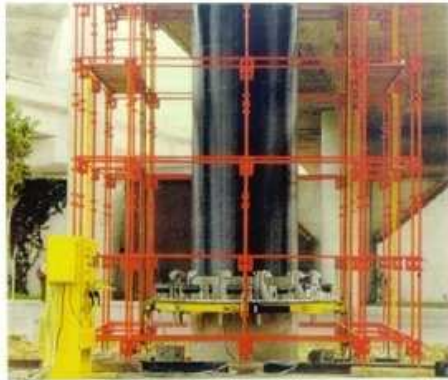
Fig 5. JACKET: Computer-Control Robot wraps Concrete Column with carbon fibers.
