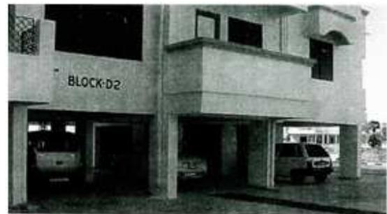
Figure 1: Ground storey's of reinforced concrete Buildings are left open to facilitate parking
