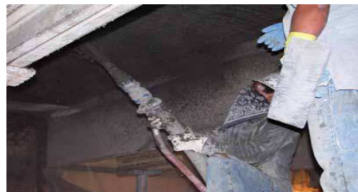
Fig.3: Application of spray-applied mortar
