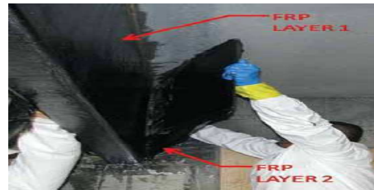
Fig.4: Application of fiber-reinforced polymer (FRP) sheet
