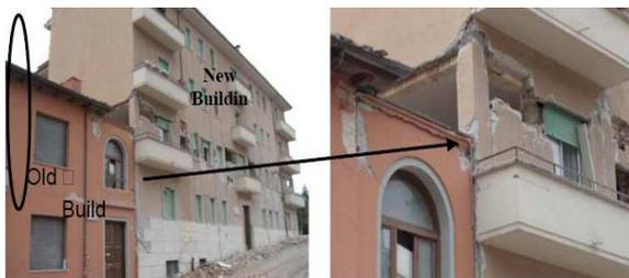
Fig 2. Pounding Between New & Old Building During 6 April 2009, Aquila Earthquake.
