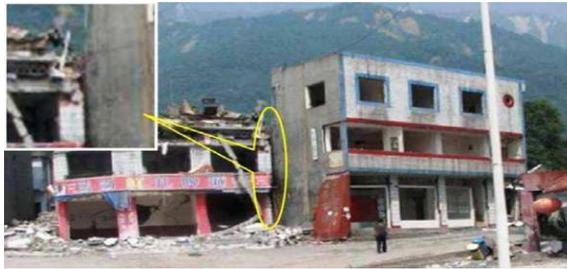
Fig 1 Pounding Occurred Between Two & Three Storey Structures during 12 DEC. 2008, Wenchuan Earthquake
