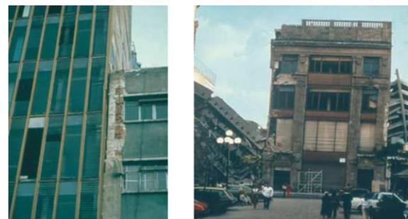
Fig. 4. Pounding Damages of Adjacent Building.
