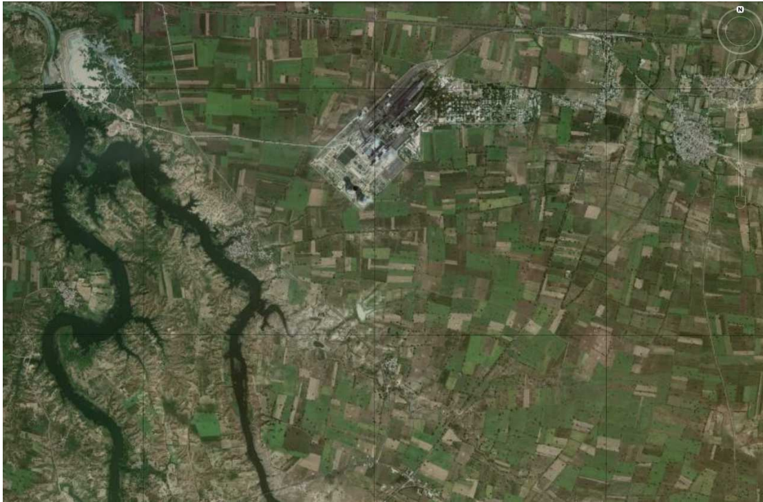
Fig.2 Satellite imagery of the Paras Power plant located in Akola district of Maharashtra
