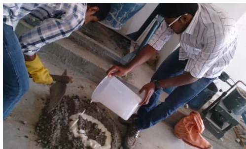
Fig – 1 Mixing of Geopolymer Concrete
