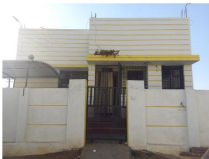
Fig. (a) - Existing Building at Akola
