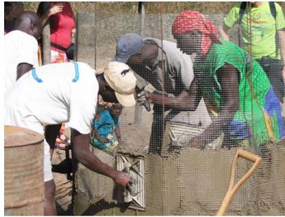
**Fig.4 Press Fill Method**
