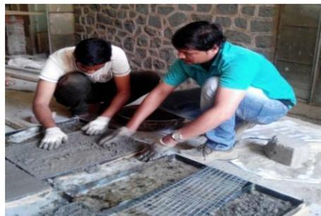
**Fig.5 Lay-up Technique**
