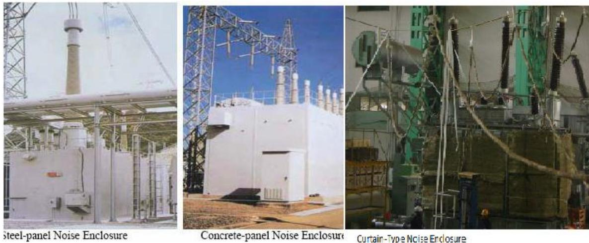
**Fig. 3.2. Different Types of Enclosures**
