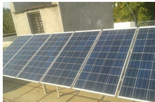
Fig.7: Erected Solar Panels Placed on Terrace
