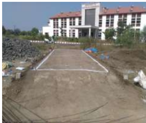
Figure 5. Combined Artificial and Composite Subgrade of Model Flexible Pavement
