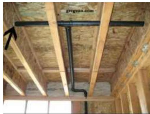
Figure 2: Pipes through web of beams
