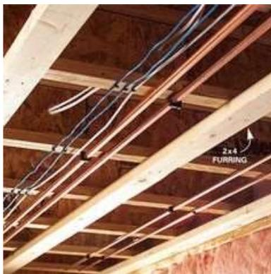
Figure 1: Service cables and pipes under beams
