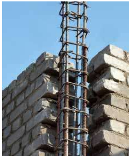
Fig. tothing at the wall to tie column interface.
