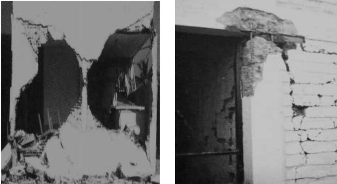
**Figure 8. Damage to confined masonry buildings in the 1985 Lolleo, Chile earthquake<sup>1</sup>**
