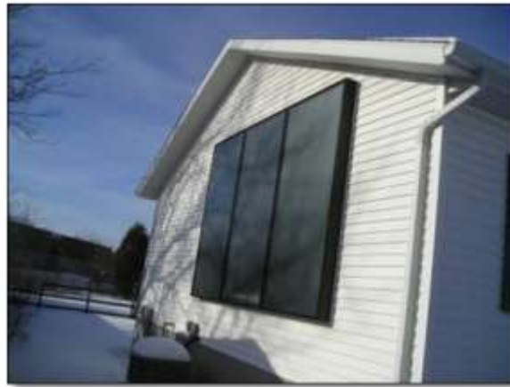
Fig 2: SPF Solar Air Heat Collector
