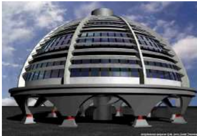
Figure 3 : Shape optimized for Seismic Energy dissipating devices and mitigating torsion effects
