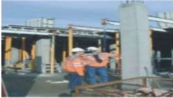
Green concrete columns
