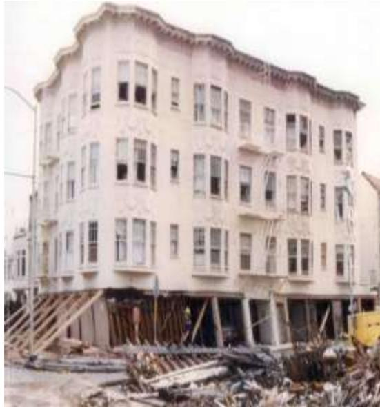
Fig 3: Collapse of Multi-Storey Building Due To Soft Storey.
