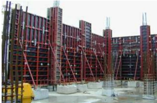
Fig. 3: Steel Formwork[9]
