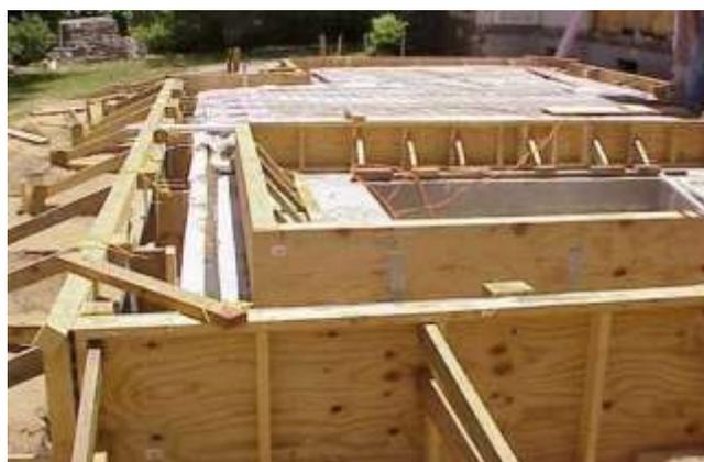
Fig. 4: Plywood Formwork[10]
