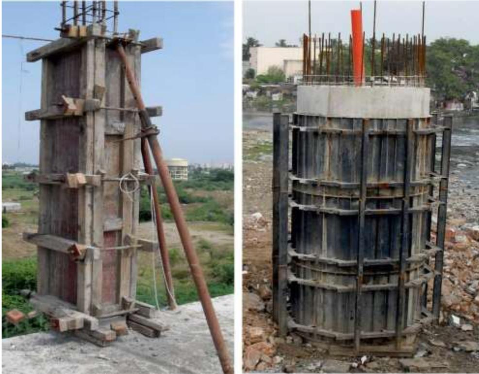
Fig. 1: Conventional Formwork System[7]
