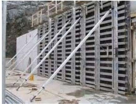
**Fig. 5: Aluminium Formwork[11]**
