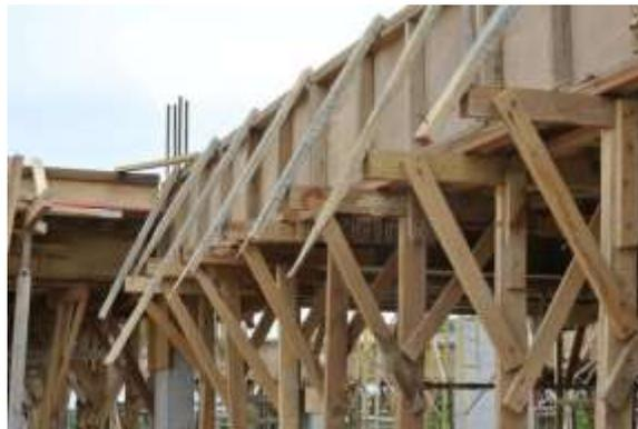
Fig. 2: Timber Formwork[8]
