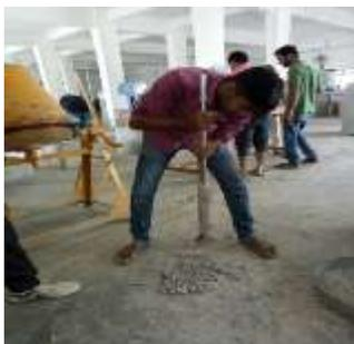
Fig.11 Crushing of Concrete Rubble
