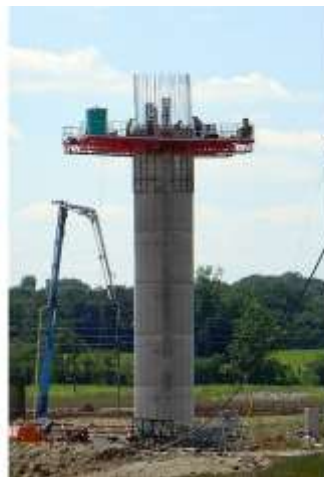
Fig. 1: Column Formwork [4]
