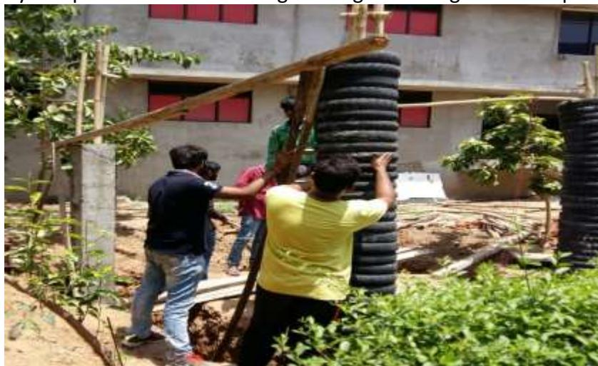
**Fig. 2 Scrap Tire as a Permanent Formwork for Column**
