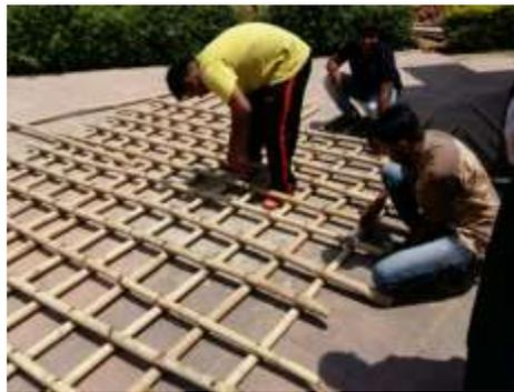
**Figure 1 Bamboo as a Slab Reinforcement**
