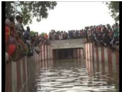
Figure: 3 underpass (source: https://i.ytimg.com/vi/_MNgGrJygd0/hqdefault.jpg )
