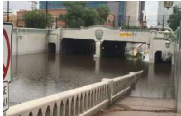
Figure: 4 underpass (source: https://mediaassets.kgun9.com/photo/2016/08/09/StoneUnderpassshotsize_1470767150258_43996236_ver1.0_640_480.JPG )
