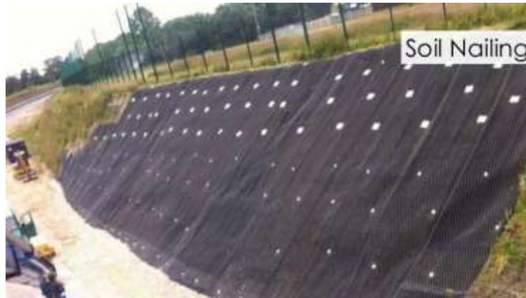
Figure 1 Soil Nailing<sup>[2]</sup>
