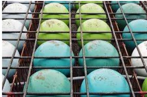
**Fig. 2 BUBBLE DECK SLAB**
