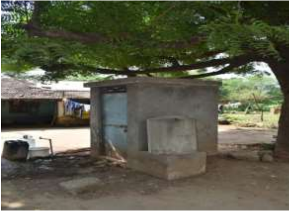
Fig. – Sanitation facility
